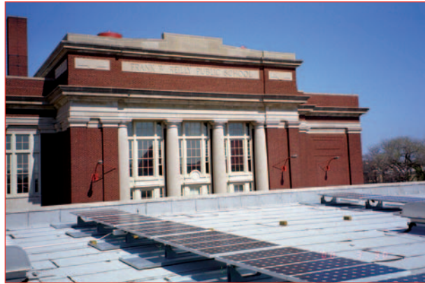
Reilly Elementary School (Chicago, IL) installed a 10.2-kilowatt solar-electric system.
