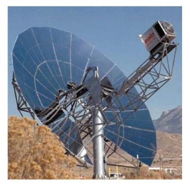
The Advanced Dish Development System is a 10 kW water pumping system developed by WG Associates for use by Native Americans in the southwest U. S.
