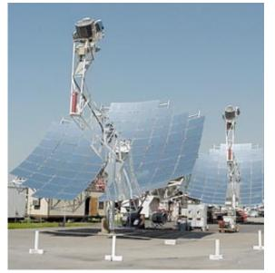
The Boeing/Stirling Energy Systems DECC project will evaluate the performance of the "critical" parts of the Stirling engine and develop the nextgeneration of the 25 kW Dish-Stirling System.
